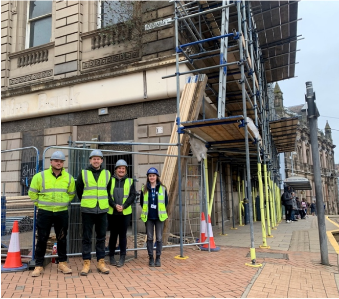
Left to right: Arron Rose , Site Manager, Andy Hare , Construction Manager, and Amy Stamford , Commercial Manager from Pinnacle Conservation and Rebecca Sleight , Senior Building Surveyor from Rider Levett Bucknall
